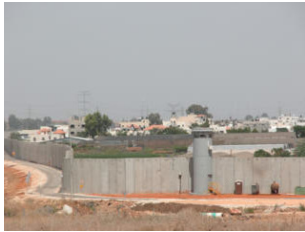
photo from: http://www.elca.org/middleeast/wall/
